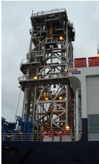
Figure 2.15: Module handling tower on RLWI vessel
