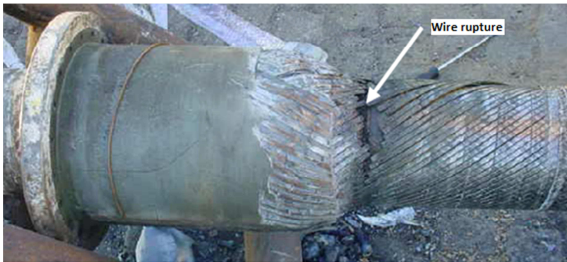
Figure 9 - Tensile armour wire rupture due to fatigue [14].
