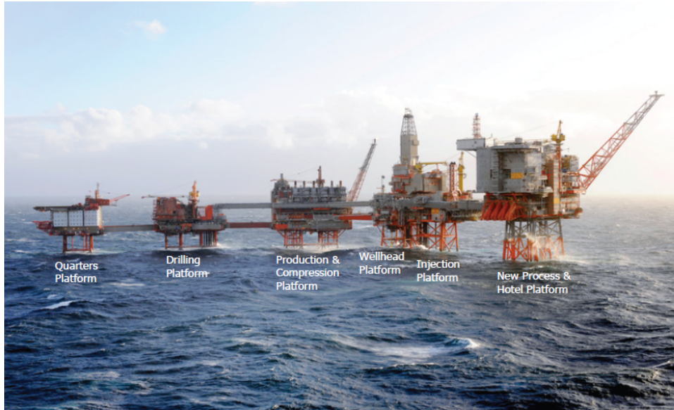
Figure 2.2: Valhall field location. The crestal part of the field consists of six platform [5].
