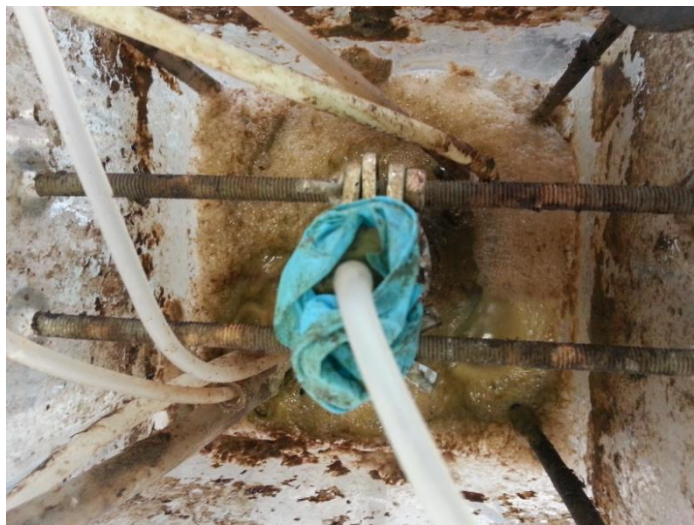
Figure 4.22: Foaming in tank C3 (Day 95)
