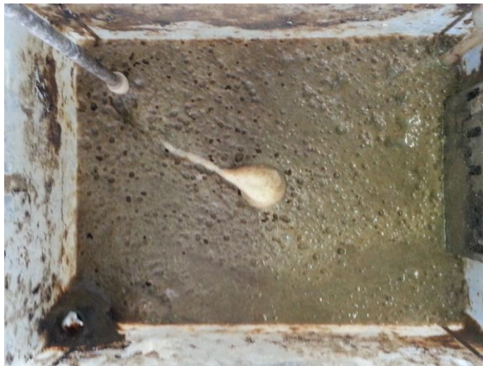
Figure 4.21: Bulking sludge in tank C1 (Day 95)
