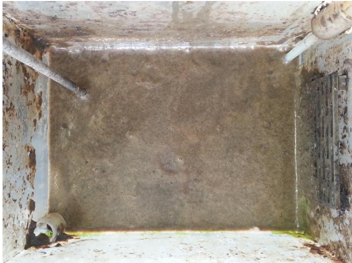
Figure 4.20: Sludge without bulking and foaming in tank D1 (Day 95)
