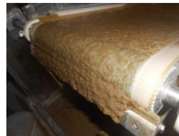
11. Filtered biofilm flocs removed by scraper to the sludge containing basin
