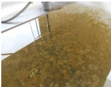
7. Pilot scale coagulation / flocculation tanks with fully formed flocs
