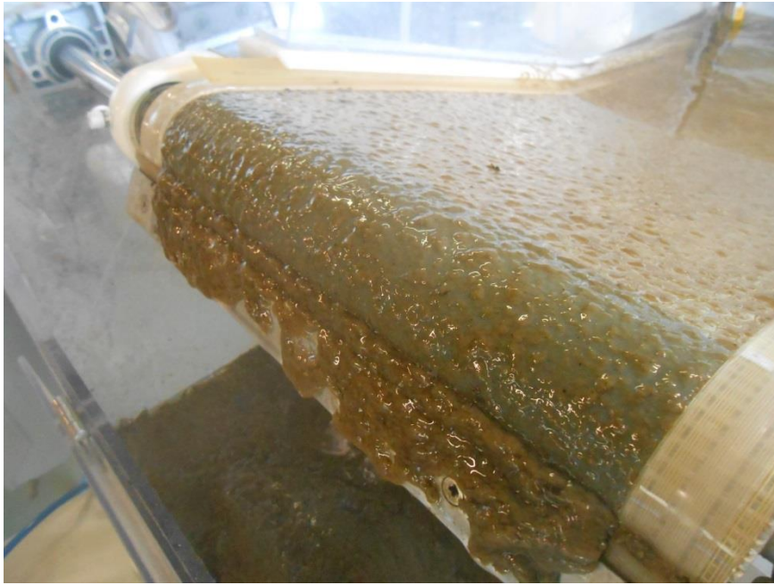
Figure 3-20: SF500 scraper removing flocculated biofilm solids
