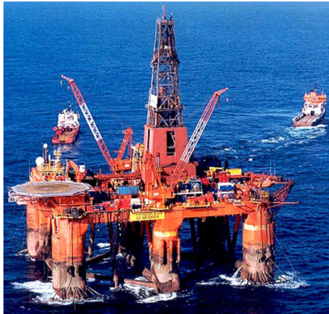
Figure 15 Transocean searcher, used for drilling the wells on Gjøa [25]
