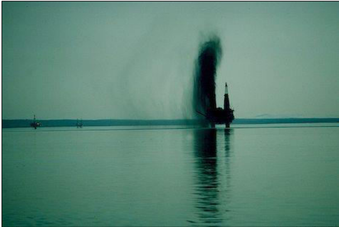
Figure 2 - Surface blowout on a drilling rig. [3]
