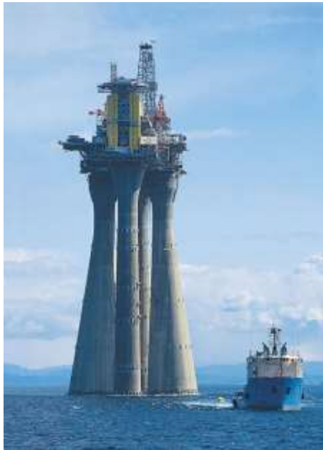
Figure 2 - Conical slipforming, Troll A
