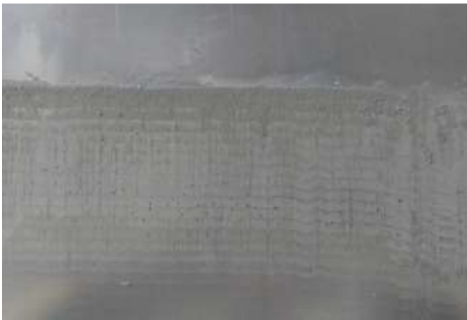
Figure 3 - Beginning growth on slipform panel
