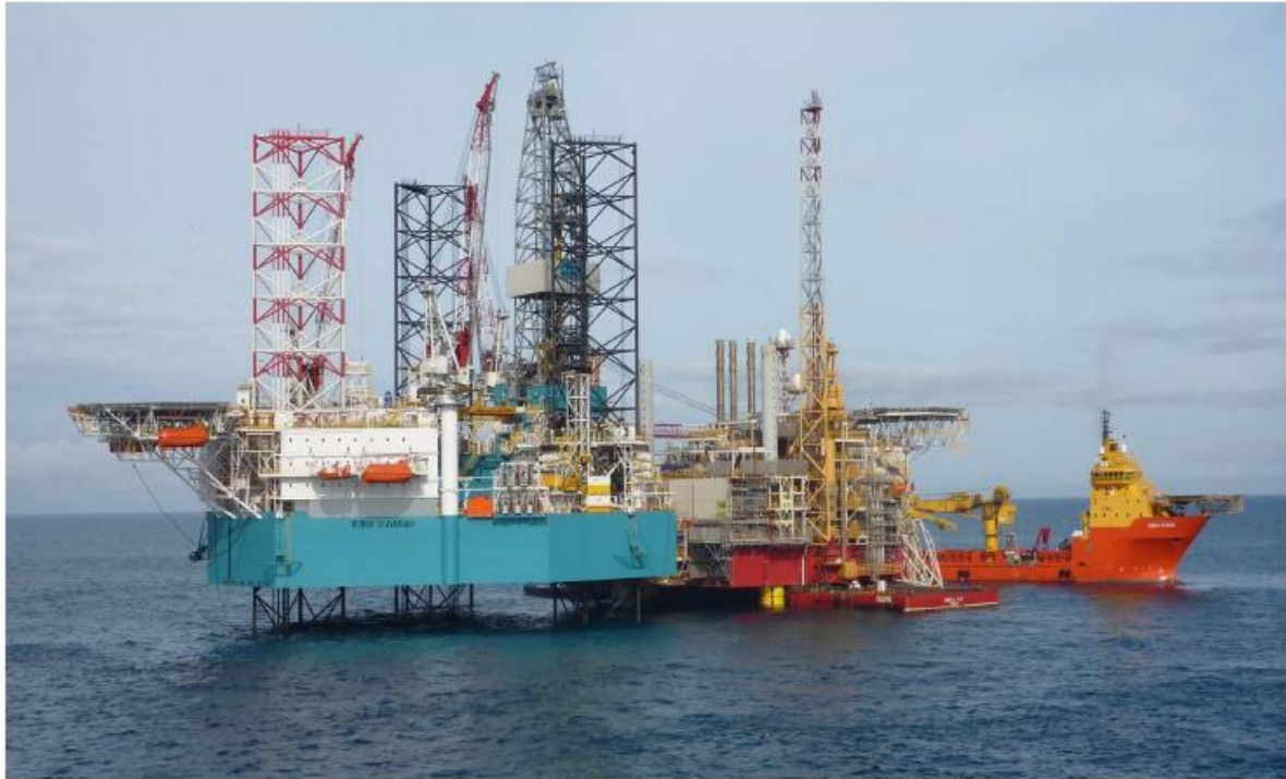
Figure 42: Yme MOPU Installation – July 2011 (Vidar, 2013)
