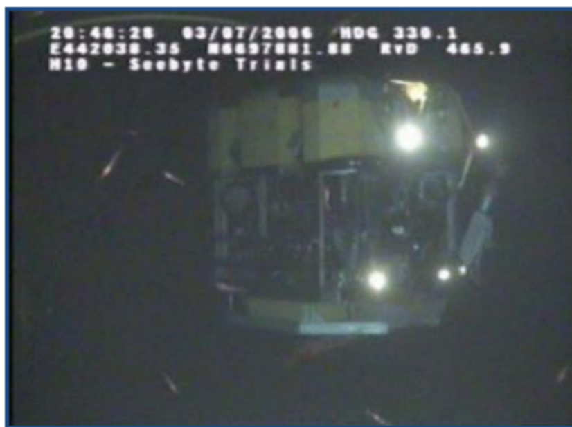
Figure 7. ROV is doing construction support [29]
