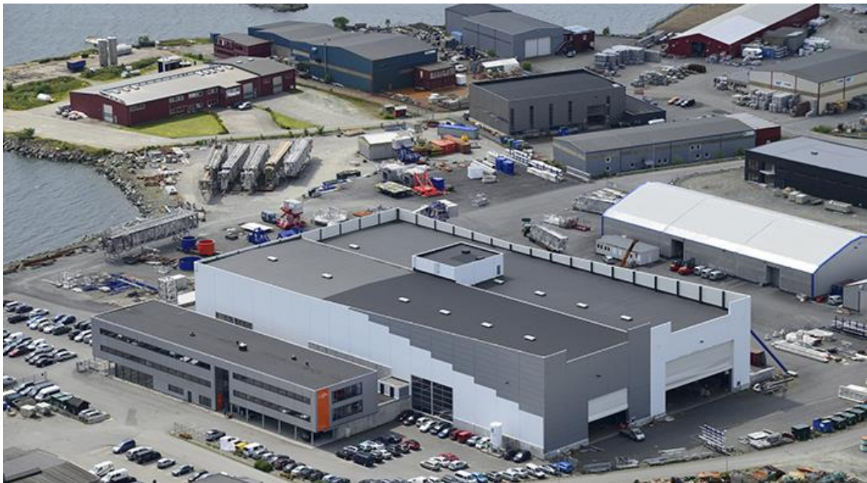
Picture 1: The main office of Marine Aluminium, Karmøy
