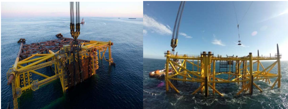
Figure 1-6 Martin Linge Jacket installation on the site
