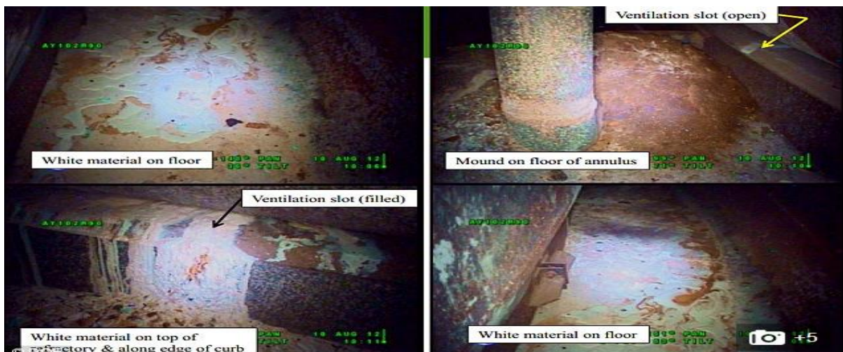
Figure 2: Pictures from the AY-102 tank between the inner and outer shells, showing the leaked liquid that has been dried into white radioactive powder. (Wilkison, 2016)
