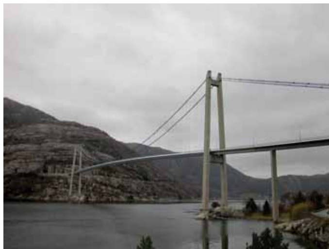
Figure A.1 South view of the Lysefjord Bridge.
