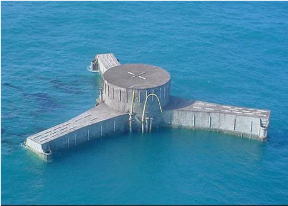
Figure 2.2 Chevron Typhoon Platform was damaged in 2005 (Ove T. Gudmestad, 2006)
