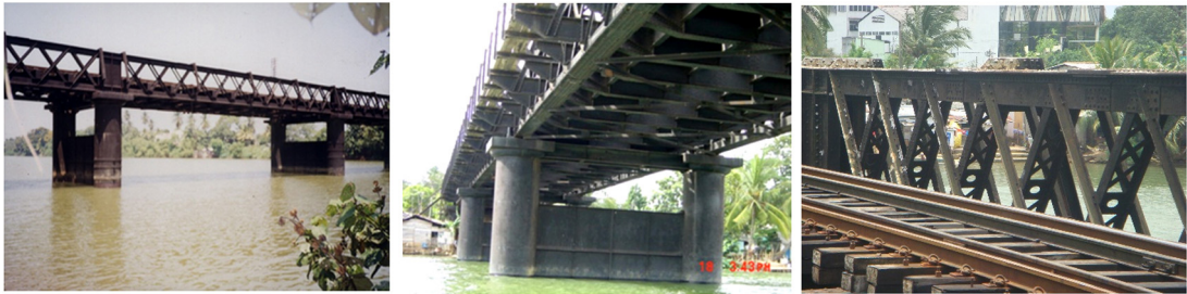
Fig. 2. General views of considered bridge.
