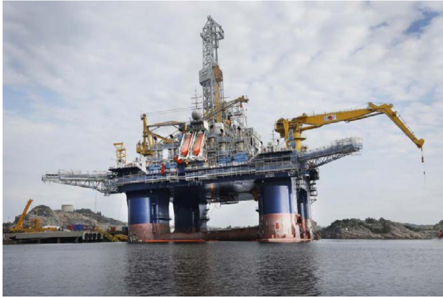
Figure 4-10: The drilling rig Island Innovator. Source; Offshoreenergytoday, (2013)
