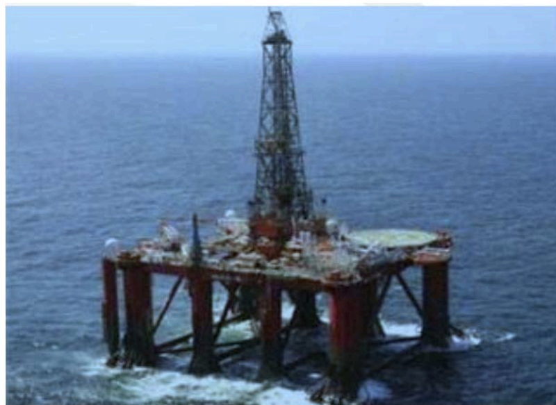
Figure 4-7: The drilling rig Aban Pearl. Source; Tinmannsvik, (2011)
