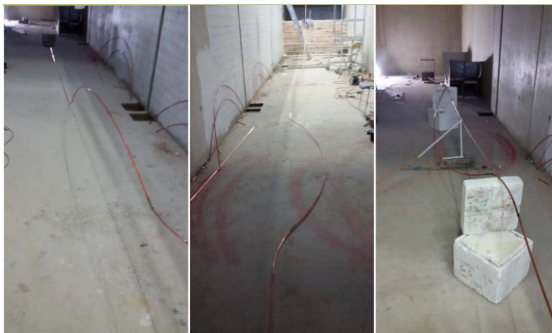
Figure 6-11: Pipe Rotation with a 3m R.C of 0.30% Residual Strain and 1-spring Pipeline Bottom Condition
