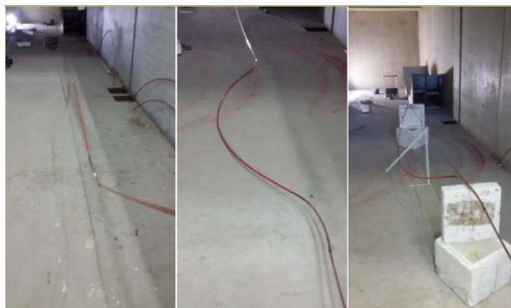
Figure 6-10: Pipe Rotation with a 2m R.C of 0.40% Residual Strain and 1-spring Pipeline Bottom Condition
