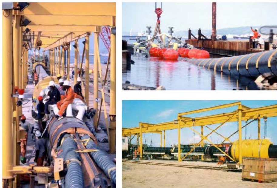
Figure 2-10: Tow installation - Pipeline ready to be towed (Courtesy of Subsea7)
