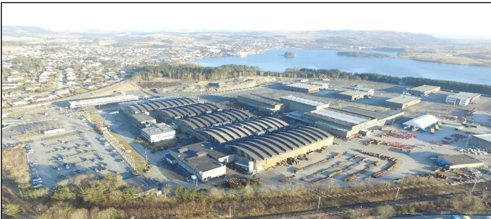
Figure 15: Picture of Kverneland Group Klepp, internal Kverneland Group photo
