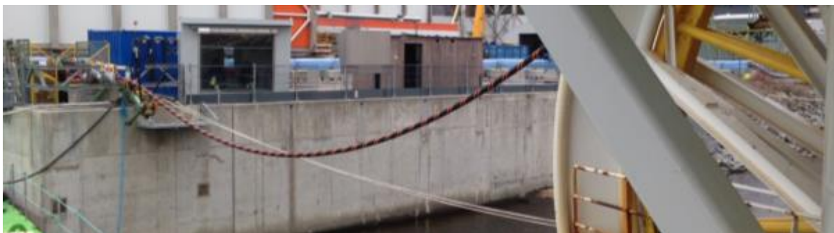
Figure 20: Cable loading to CLV (photo: Louise Våbenø).
