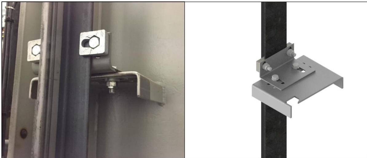
Figure 9. Guide structure of elevator cars [internal document, TK].
