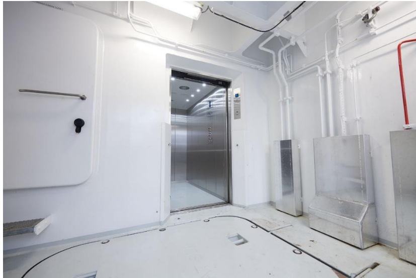
Figure 3. Car with stainless steel interior [internal document, TK].
