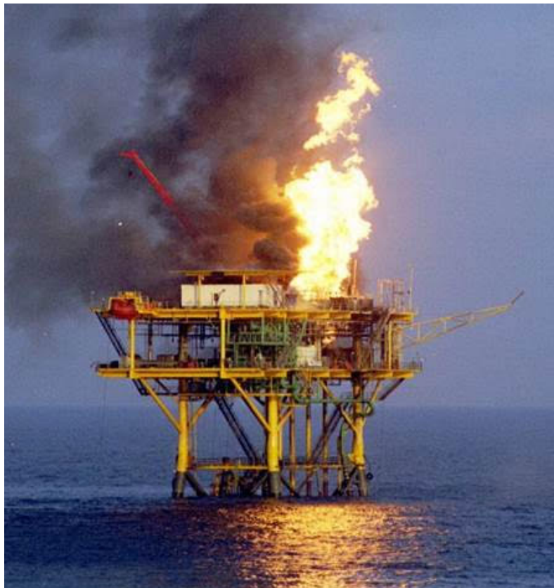
Figure 3-2: Severe incident due to poor quality well barrier [6]
