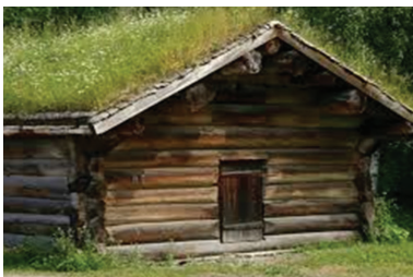
Figure 4: Old cogged house.
