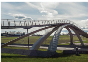
Figure 29: The da Vinci bridge, Ås, (2001).
