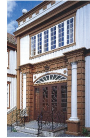
Figure 22: Leangen Imitated hewn stone.
