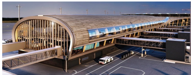
Figure 28: Oslo Airport, new pier.
