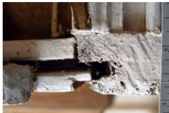
Picture 16 The wings are indicated with tongue and groove joint.
