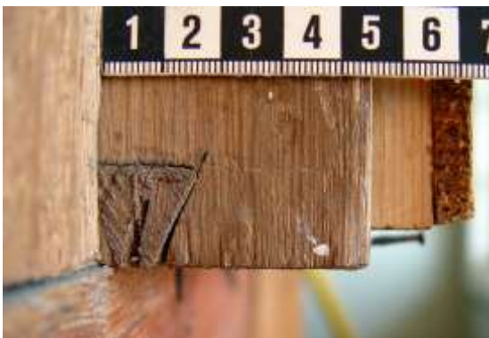
Picture 15 Dovetail joints of the frame.
