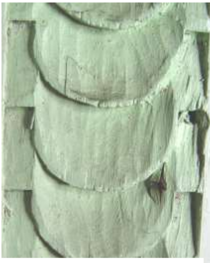
Picture 23 Detail of the carving behind the pillars. Tool marks are visible in the glazing light.
