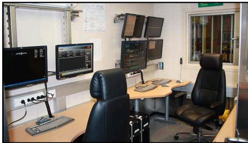
Figure 6.31: control room (Grebstad, 2014)
