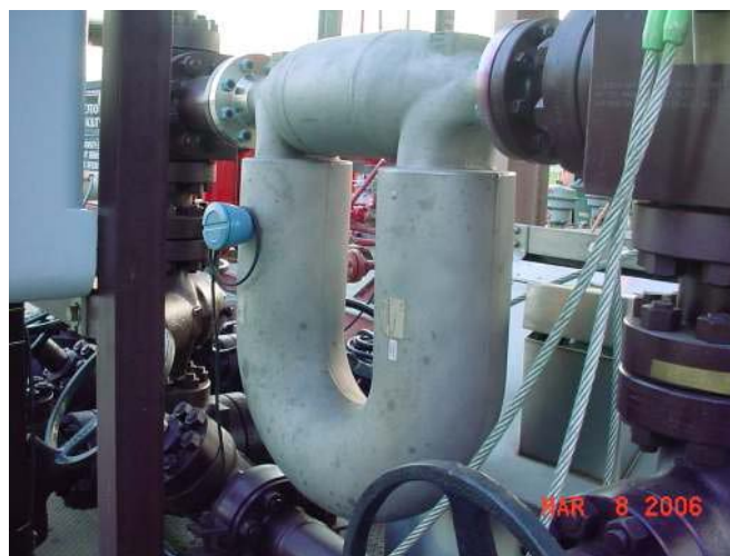
Figure 5.17: Mass flow meter (Coriolis flowmeter). (Tercan, 2010)
