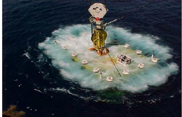
Figure 2.11: Lowering of Manifold through splash zone. (He, et al., 2012)
