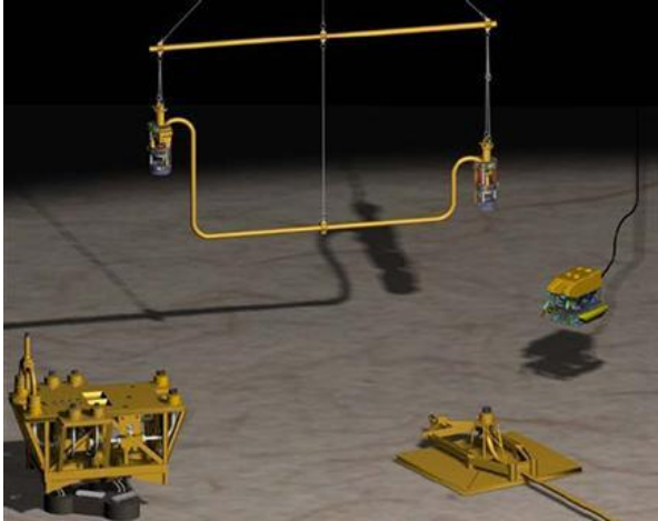
Figure 4.6: Well jumper with spreader beam. Picture provided by Equinor.
