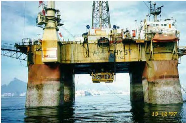
Figure 2.6: SEMI Drilling riser for installing 240Te Manifold. Courtesy of Petrobras. (He, et al., 2012)
