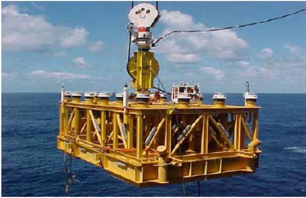
Figure 2.10: Lif-off and overboard the Manifold. (He, et al., 2012)
