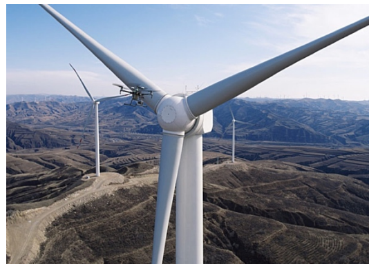
Figure 22: Drone inspection of an onshore wind turbine (AviatDrones, 2018)
