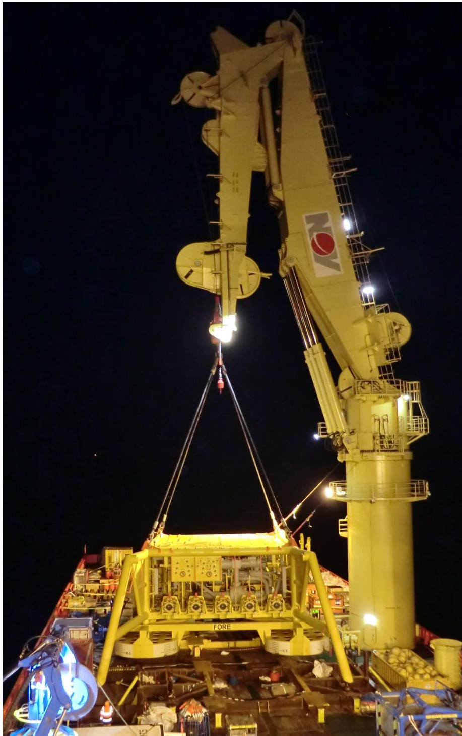
Figure 13 – Kirinskoye Subsea Manifold Lift off [4]
