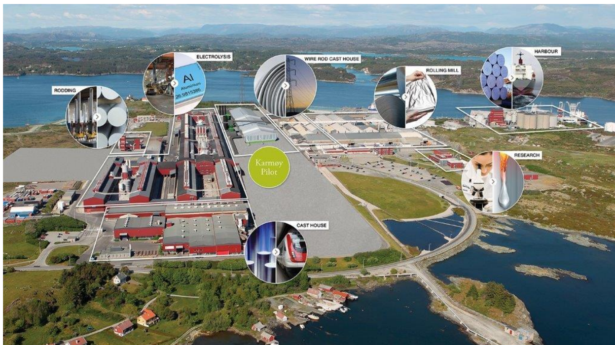
Figure 9: The aluminium plant at Karmøy and the different units located in the factory
