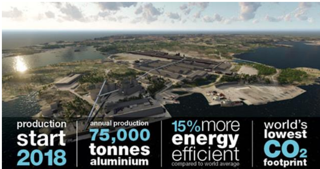
Figure 3: Characteristics of the new technology pilot at Karmøy
