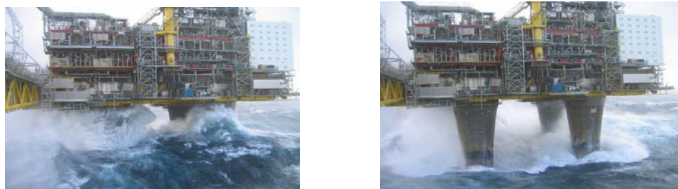
Figure 2 Waves – Major fatigue load for North Sea platforms, ref/3/
