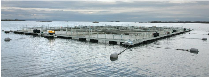
Figure 6: Illustration of a traditional steel cage consisting of four separate net pens (AKVA Group, 2017).
