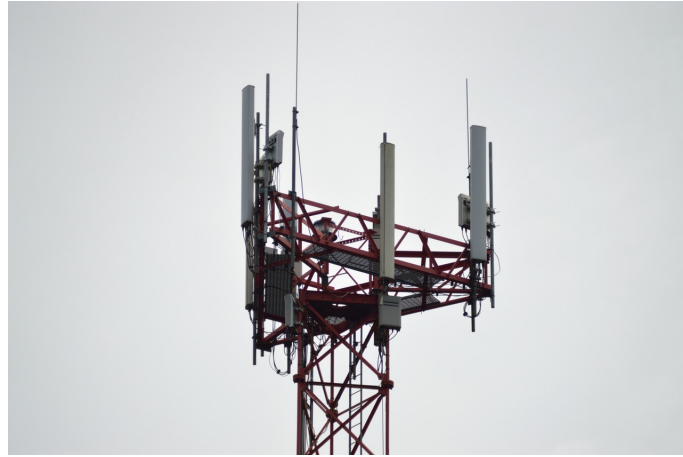
Figure 2.4: Photograph of LTE antennas placed on a tower, acting as a base station [3].
