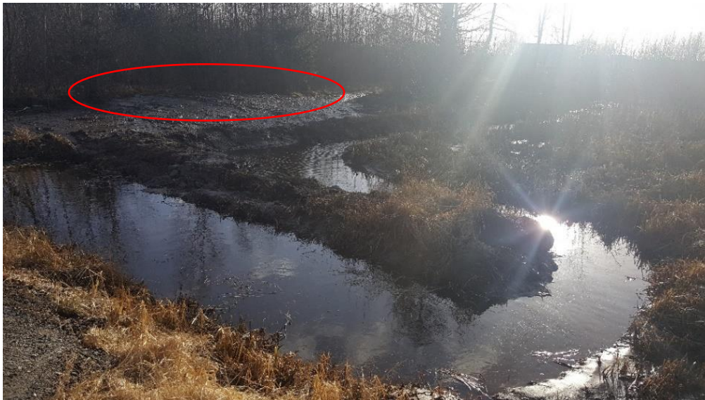
Figure 3-7 Picture of Pond 1 in Leikvollbekken after sediment removal by Stavanger municipality. Removed sediments were placed next to the wetland, marked by a red circle. (5 th of April 2018)
