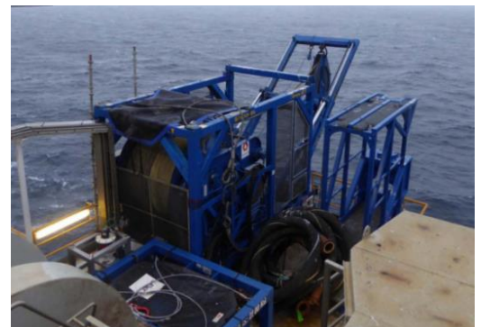
Figure 3. 6 Umbilical Winch and Hose Handling Platform on Deck [76]
