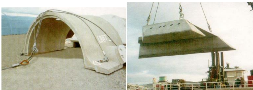
Figure 2.10: Standard concrete cover shape and its lifting operation (slp-projects.com)
