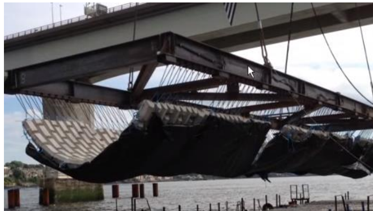
Figure 2.14: Multi-deployment frame provided by SPS ( youtube.com/sps )
