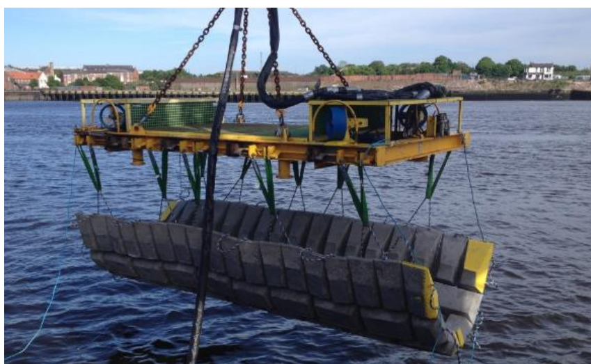
Figure 2.17: IMF during installation of a concrete mattress (deepoceangroup.com)
