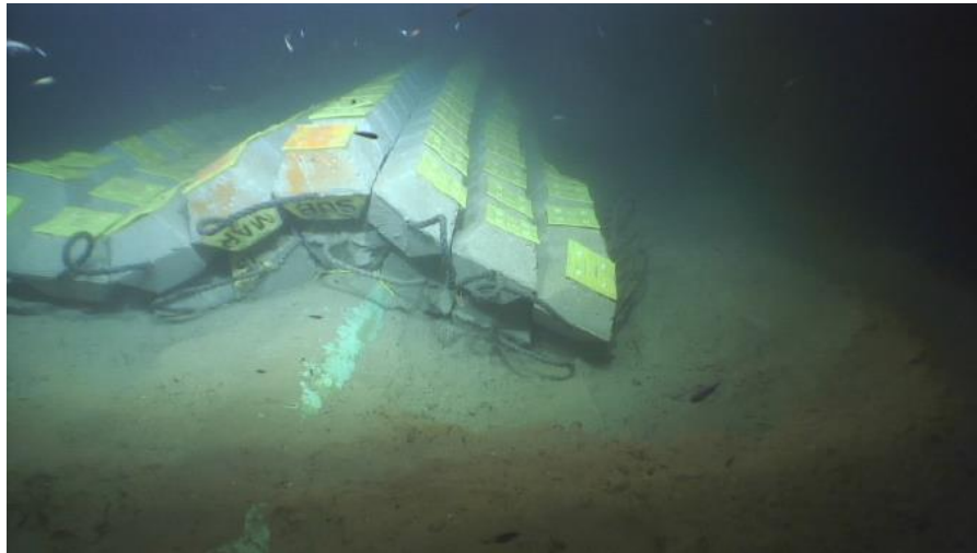
Figure 2.5: Flexible concrete mattress over a subsea pipeline (oedigital.com)
