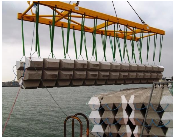
Figure 2.13: Mechanical lifting frame
