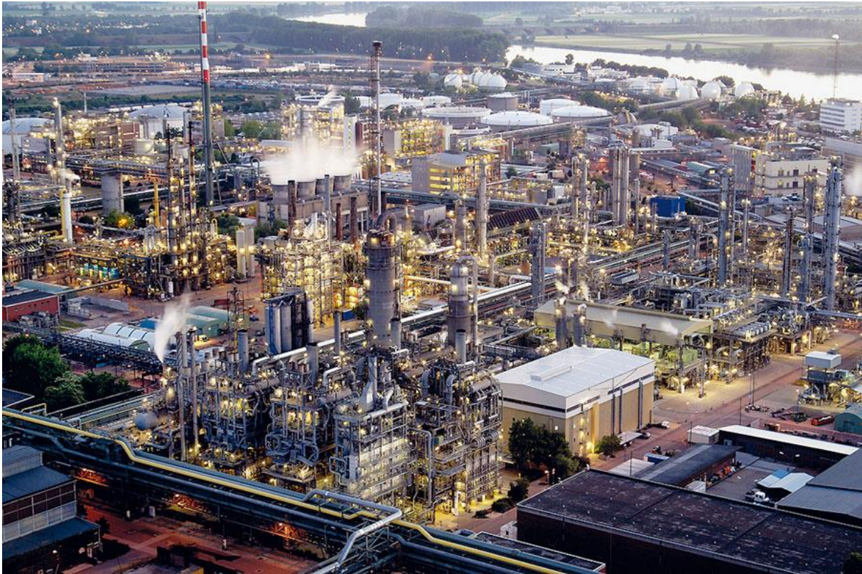
Figure 6-4 Aerial picture of part of Chemelot site
