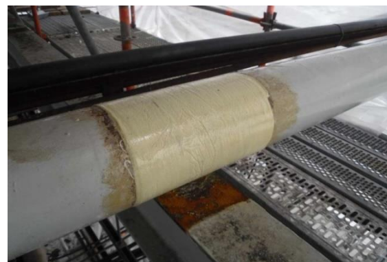
Figure 9-4 Full composite wrapping
