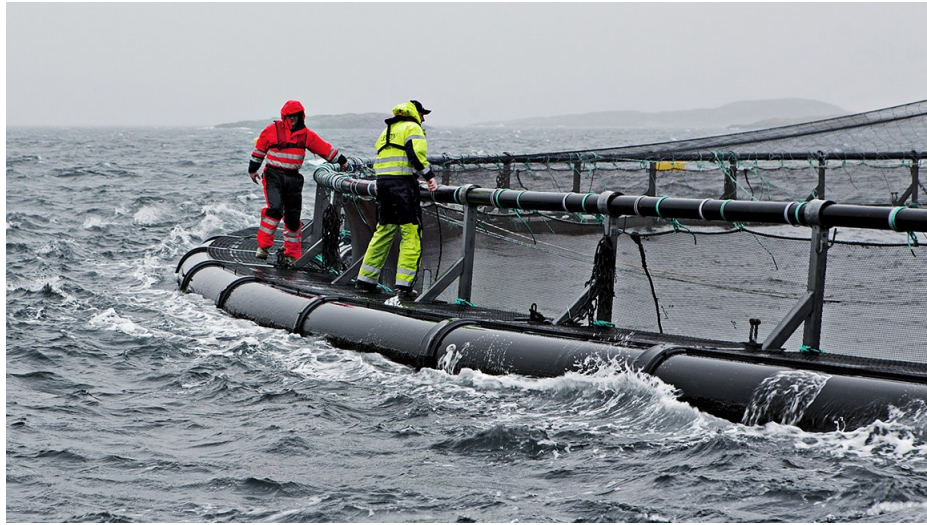
Figure 3.2: Double-pipe floating collar of a gravity-based fish cage (Source: Aqualine AS)
