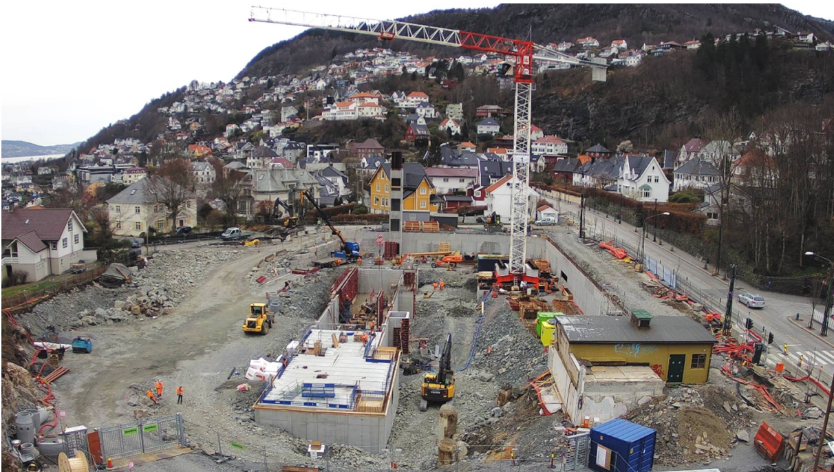
Figure 4.2: The construction site in Spring 2019. Picture provided by Skanska.
