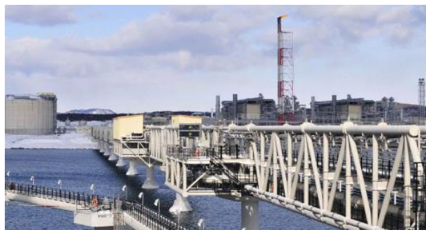
Figure 23. Tanker Loading Unit (TLU) (Photo courtesy of Sakhalin Energy Company)
