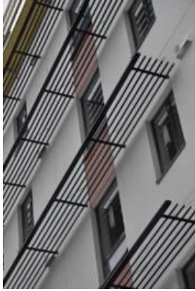
Fig.12: Solar shading with built in photovoltaic panels on the Jampankaari building (Nieminen, 2011, p.16)
