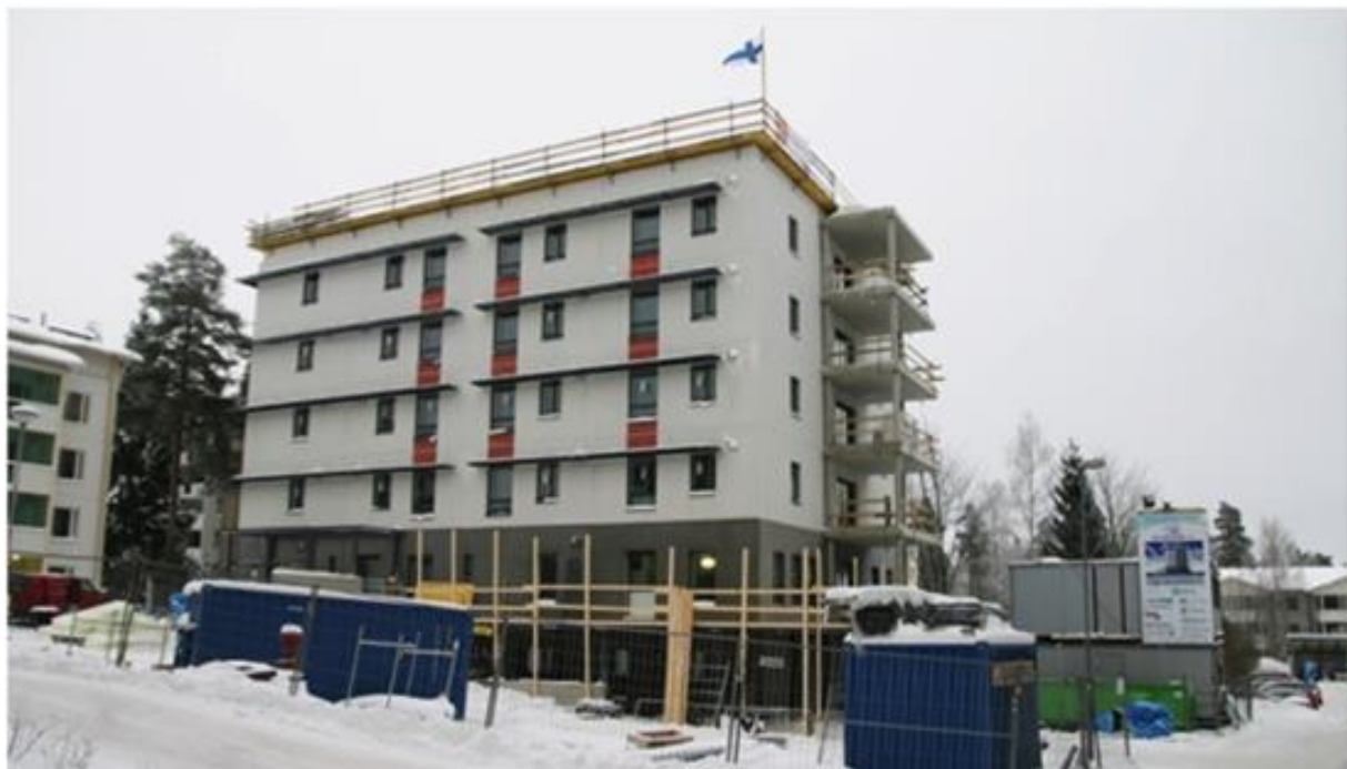
Fig.9: Jampankaari zero energy house under construction #1 ( Vallox.com, 2019 )
