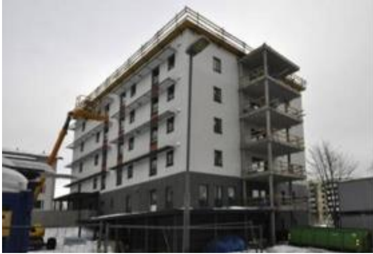
Fig.10: Jampankaari zero energy house under construction #2 ( Vallox.com, 2019 )
