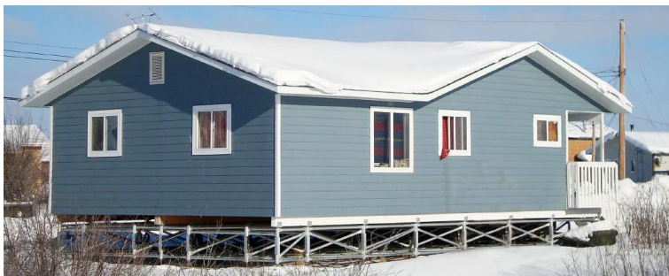
Figure 14: A typical Multipoint Foundation (Rognved et al., 2017).
