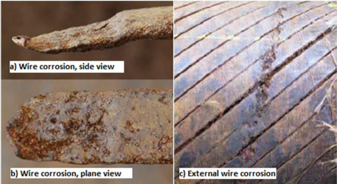
Figure 57 Shows corroded tensile armour wires due to a breach of outer sheath [19]
