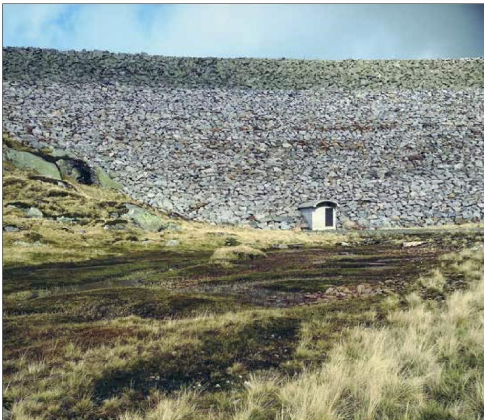
Dam at Roskreppford
