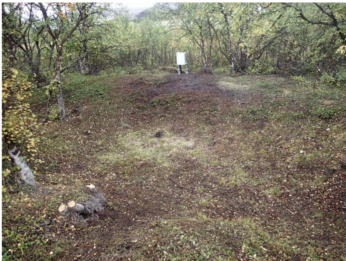
Figure 26: Overview of the site, after the field work and installation works. White cabinet: Datalogger BioForsk. Hypnos is located behind this cabinet. The trench is located underneath the greener turfs amidst the brown area. Photo: MVH Consult.
