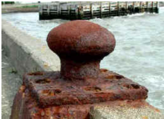
Figure 4 - Uniform attack [8]
