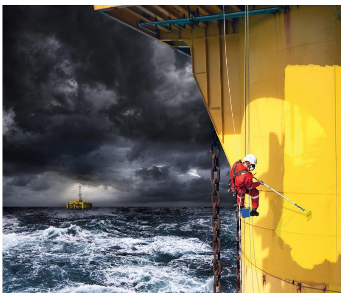
Figure 19 - Paint coating [28]
