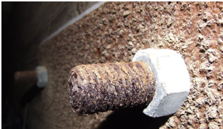
Figure 5 - Galvanic corrosion [11]
