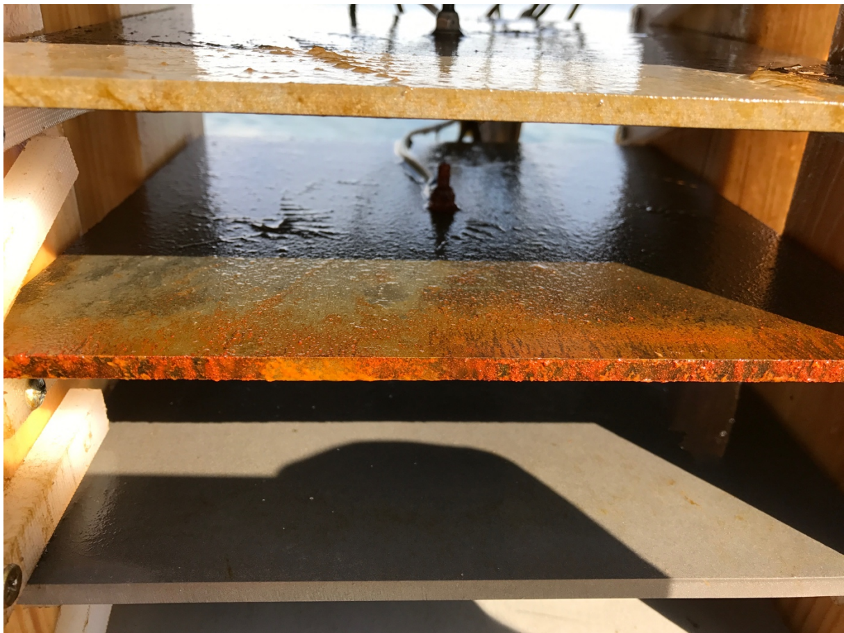
Figure 45 - Corrosion on the steel cathode in system 1
