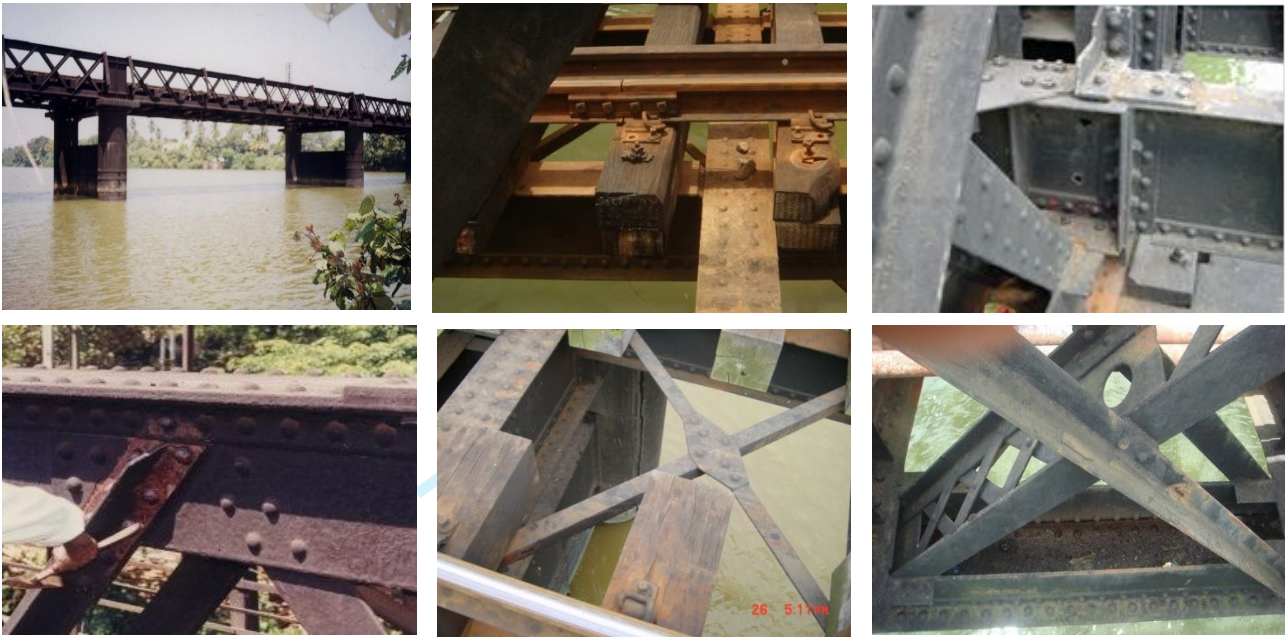
Fig. 6. General view and some of the corroded locations of the bridge 4
