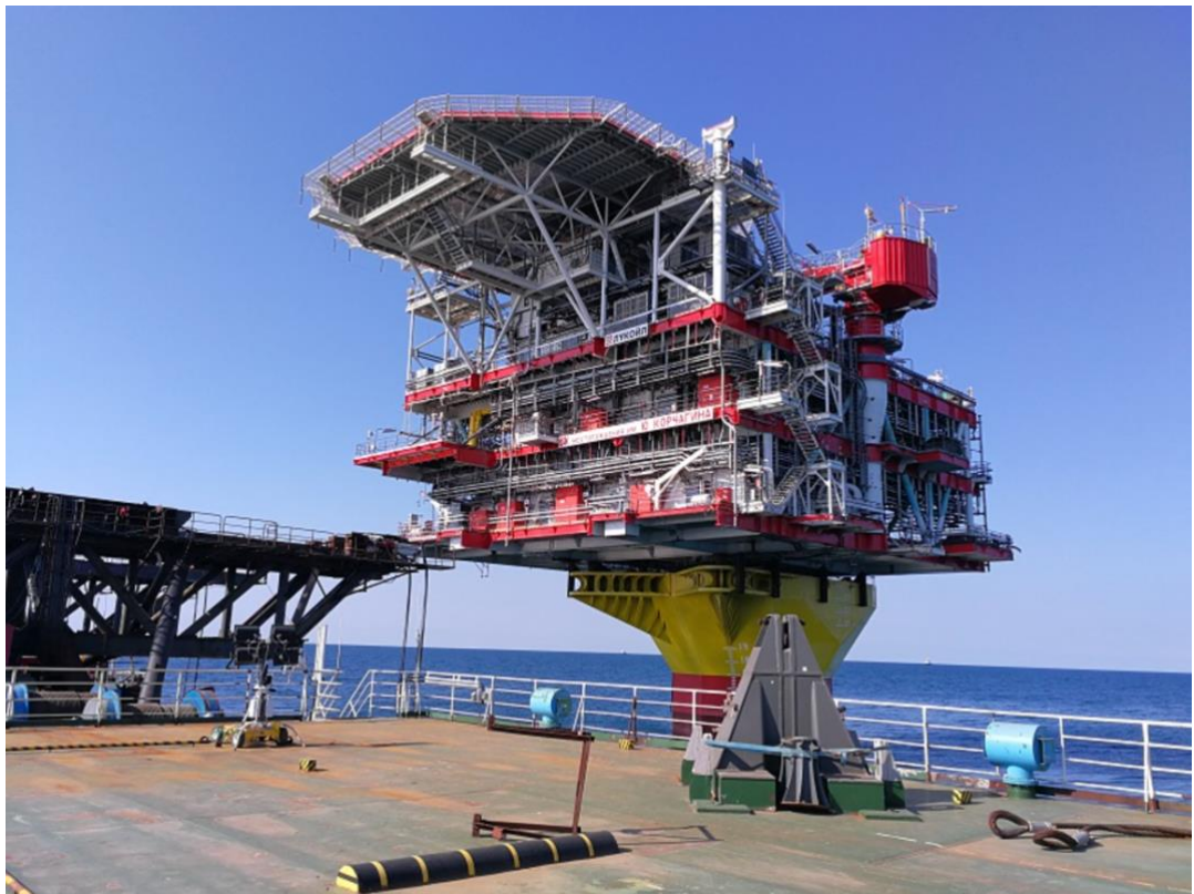
Fig. 2.12 Upper part of the satellite platform [22]
