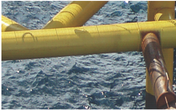
Figure 1.2: Tubular joint with loaded chord member.
