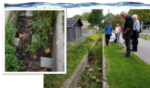
Figure 19 – Stormwater chute (Oslo Kommune Vann- og avløpsetaten, 2016) The chute has small blocks which slows the runoff water down.
