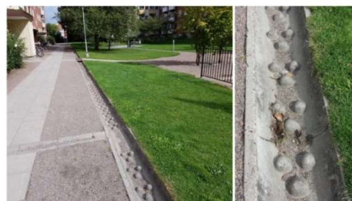
Figure 20 – Stormwater chute (Oslo Kommune Vann- og avløpsetaten, 2016) The chutes have small bumps to slow down the water and increase oxygen level in the water
