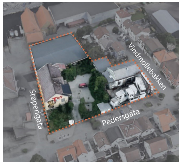
Figure 13: Previously project site
